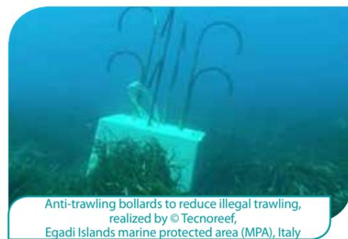
Anti-trawling bollards to reduce illegal trawling, realized by © Tecnoreef, Egadi Islands marine protected area (MPA), Italy
